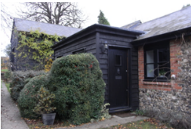
Barn conversion – Green End
